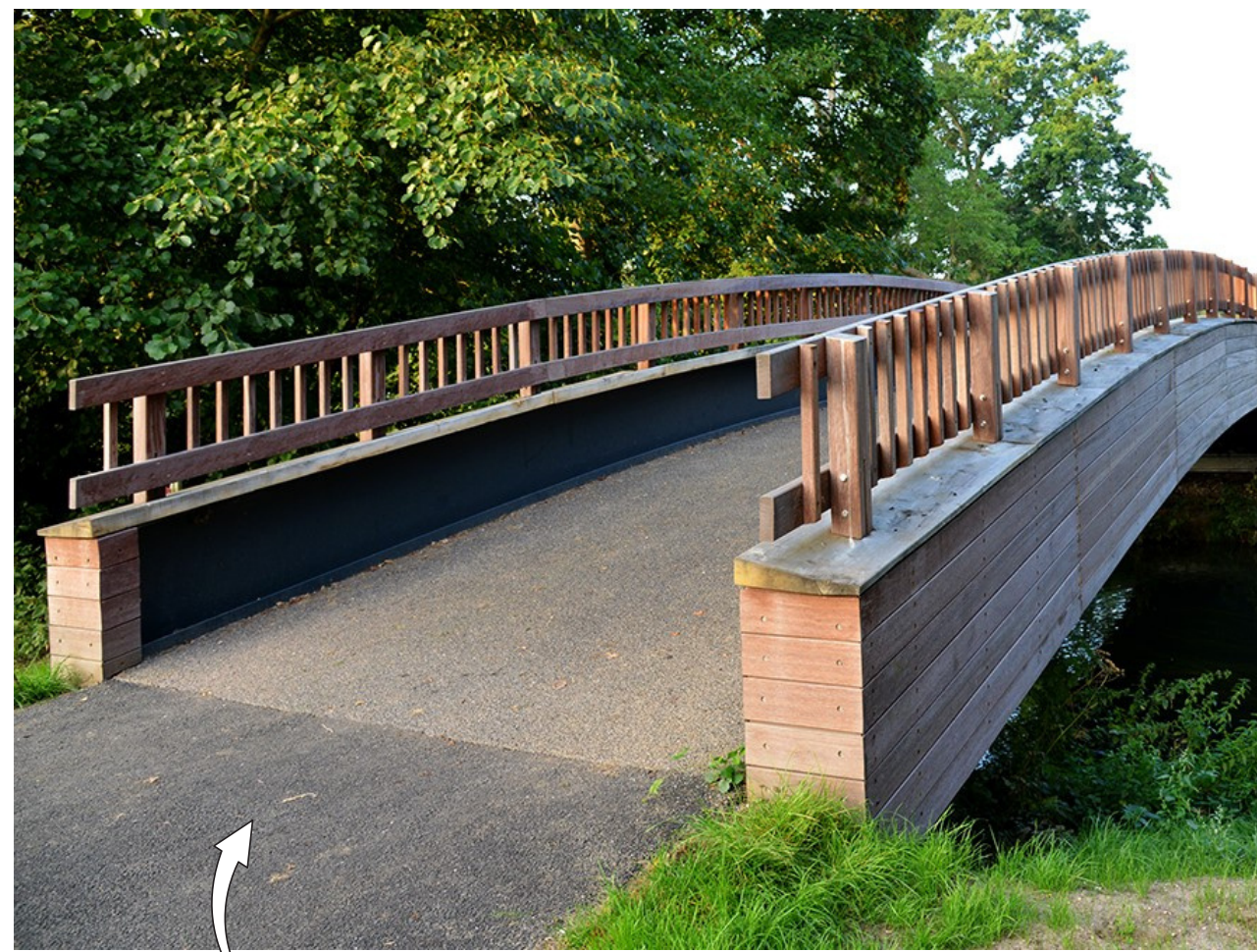
Shallow arch with graded crossing
